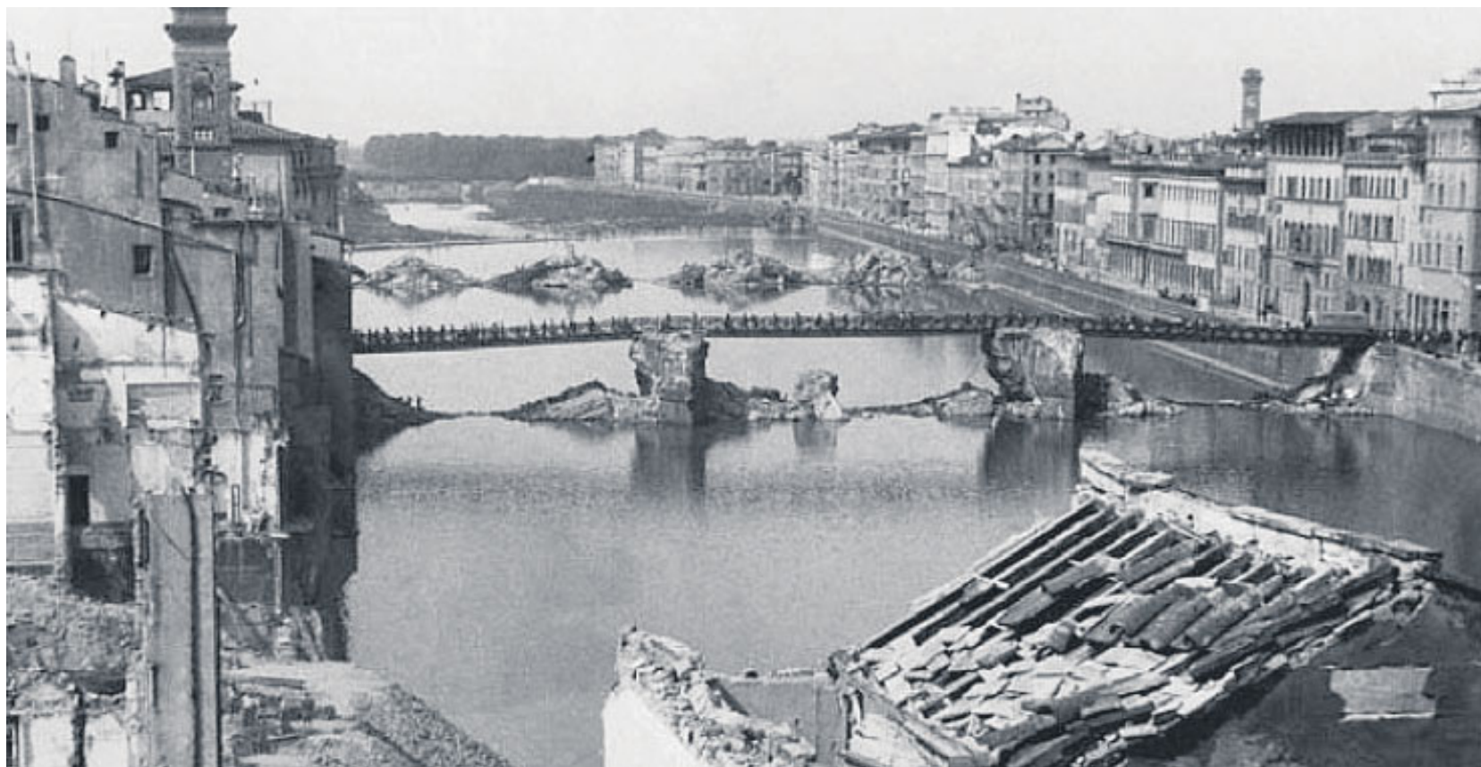
Si noti la passerella gettata sui pilastri rimasti in piedi del Ponte Santa Trinita a Firenze PENNOYER PAPERS, DEPARTMENT OF ART AND ARCHAEOLOGY, PRINCETON UNIVERSITY
